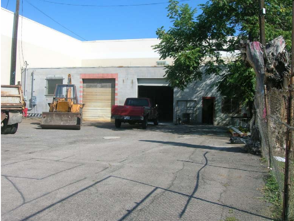
Front view of site from 700 South
